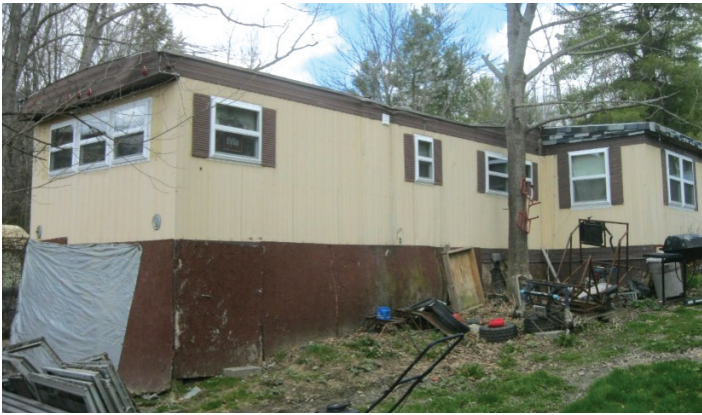
This mobile home just received window replacements through the Weatherization Assistance Program administered by Tioga Opportunities. The residence is in a condition typical of many Broome County mobile homes, yet is still in need of skirting, roofing, and other repair work.
